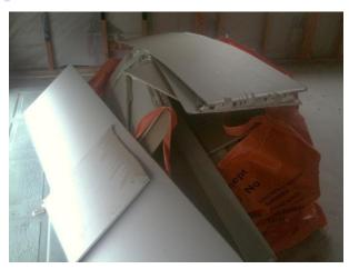
Their process was to unwrap and assemble the flexibin as early as possible in the process, and deposit offcuts in it as they went. This created a potential tripping hazard in the garage, and proved to be 'an annoyance' to the installers, particularly as they came to install the plasterboard in the garage and had to work around the unit. Their solution was to install plasterboard in the garage first, which partly alleviated their concerns.
