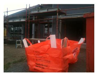
The other installers (for Stonewood and Jennian) quickly concluded that filling the bin progressively throughout the installation was not desirable, and so instead left offcuts in each room as they installed.
