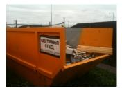
Transpacific provided a 'Flexibin' system, consisting of a proprietary polypropylene bag. This was provided to installers as a small handheld folded bag that could then be assembled into a two or three cubic metre unit for receiving waste plasterboard. A customised gantry truck was employed by Transpacific to facilitate pick up of these units.
